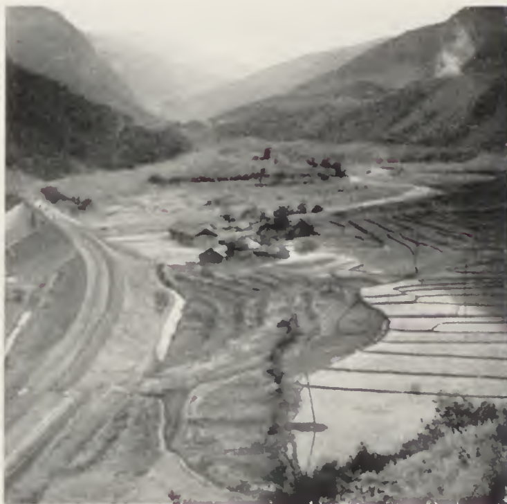
Rice fields in a mountain valley on Firouzkuh-Shahi road. The new trans-Persia Railway in left foreground.
